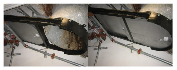
**<u>OPEN POSITION</u>** (STANDARD SETTING) Both Doors Are In Open Position **CLOSED POSITION (@ CONTAINER CHANGING)** Manual Door Only Is Closed Using Handle Fusible Link Does Not Have To Be Removed!
