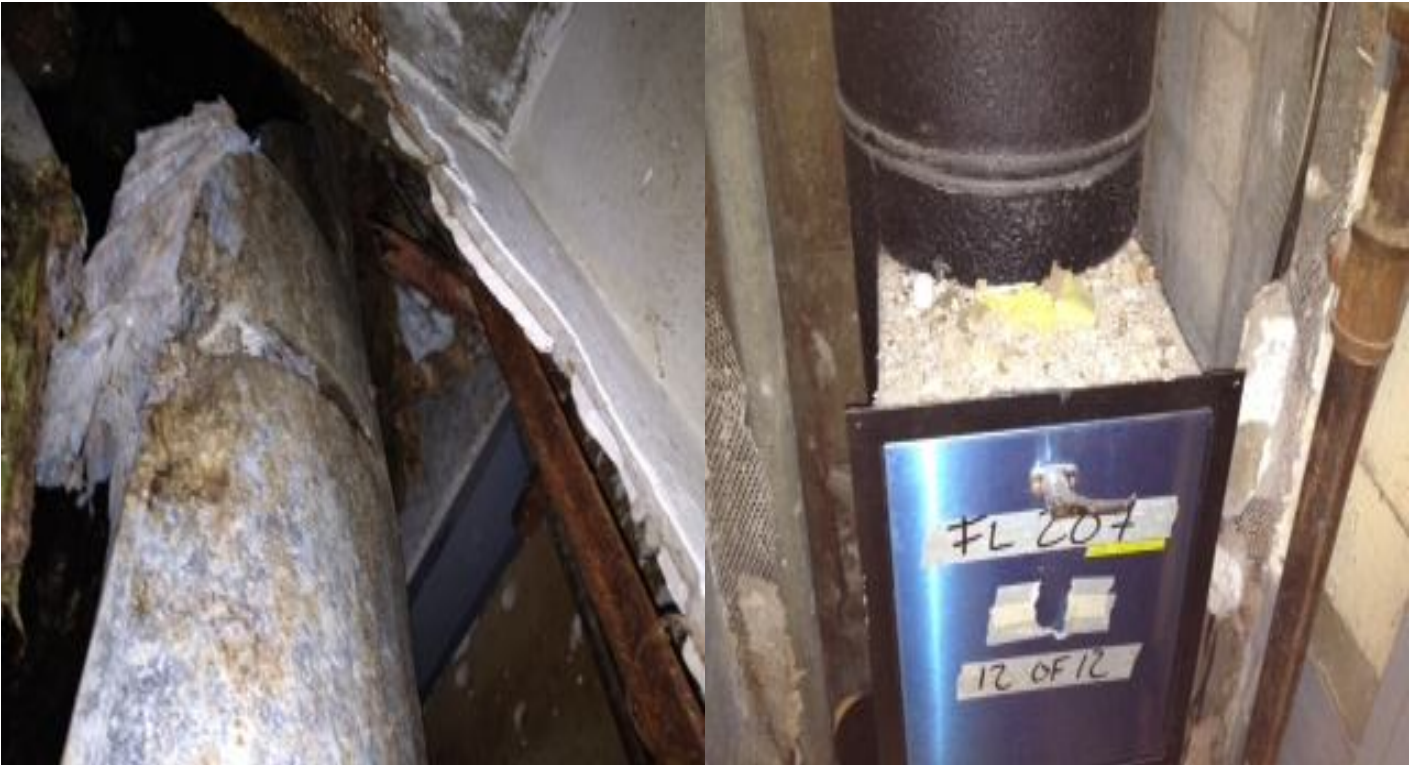
EXISTING "TORN APART AT SEAMS" CHUTE
