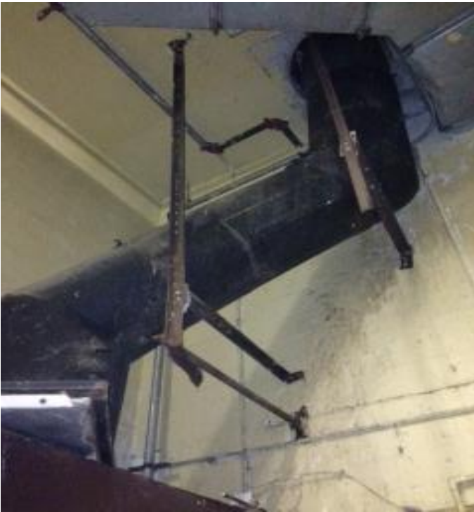
45 DEGREE CHUTE W/ CLOGGED OFFSETS
