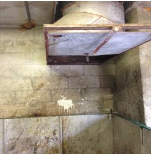
WALL SPLATTER (CHUTE TOO HIGH)
